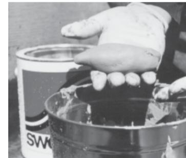
Fig. No. 2: For active water leaks, mix HydraPlug into a heavy putty and form into a plug for holes or a rope shape for cracks.
