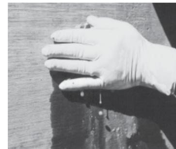
Fig. No. 3: When HydraPlug begins heating up, force into hole or crack in one swift movement. Keep pressure applied without disturbing for three minutes.
