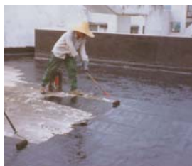
PRIOR TO COATING
